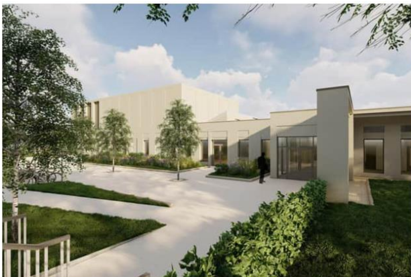
Artist's impressions, subject to further design development and planning approval. ©2024 West Northamptonshire Council and pHp Architects.
